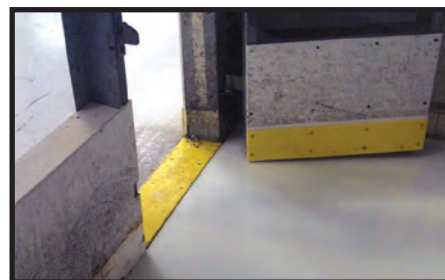
Synthetic ice installed on floor of players' box.
